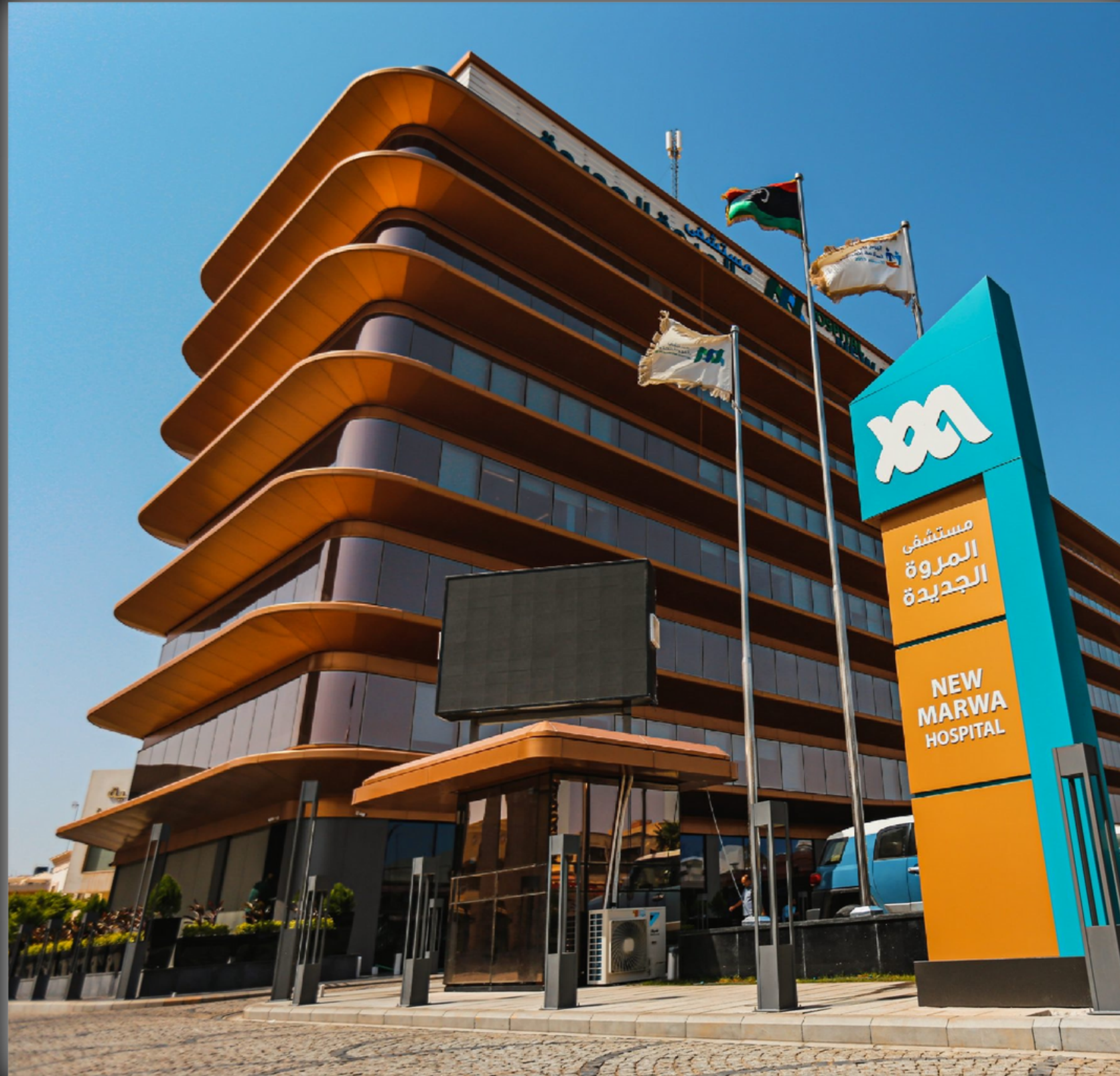
New Marwa Hospital - Benghazi, Libya.
